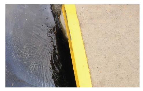
Figure 1. Typical runoff from a parking lot going into a storm sewer. Notice that traces of oil are visible to the naked eye. There are many other pollutants in parking lot runoff such as various metals, sediment, salts, and litter. *Photo by Susan Day.*
