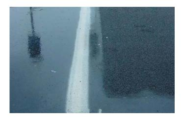
Figure 18. A comparison of traditional asphalt (left) and porous asphalt (right) when wet. The gaps created by leaving out the finer particles in porous asphalt allow water to infiltrate pavement and into the structural soil reservoir below. As a result, porous asphalt appears dull when wet, because water runs through and does not pond, which creates a high friction surface. *Photo by Ted Haffner.*
