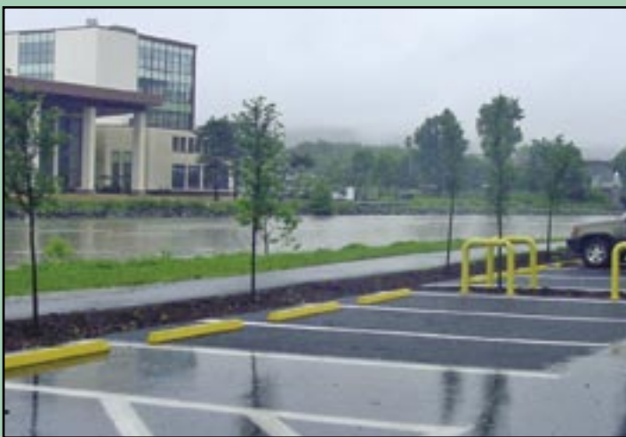
This is a 14-car parking lot in the city of Ithaca entirely built on 24" of CU-Structural Soil. In this rainy picture you can clearly see the traditional asphalt as it looks slick from the water running off it compared with the porous asphalt, which looks dull as rainwater goes through its surface. Subsequent to this construction, areas of both types of asphalt were cut out and elm trees were planted.
