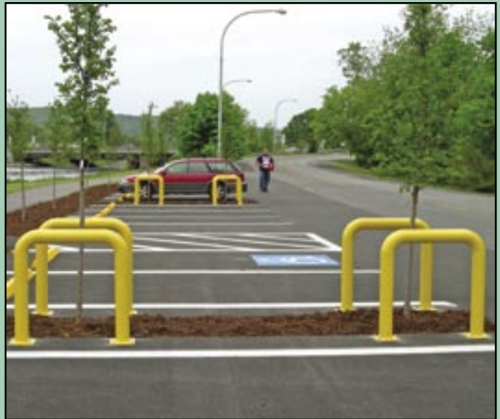
Here is the Ithaca, NY parking lot in the first year after planting. 'Accolade' elms were planted in the porous asphalt and traditional asphalt. Both surfaces have CU-Structural Soil underneath. We will be evaluating the growth of all trees in both surfaces over time.
