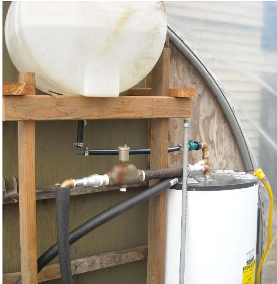
Under bench heat with electric hot water heater
