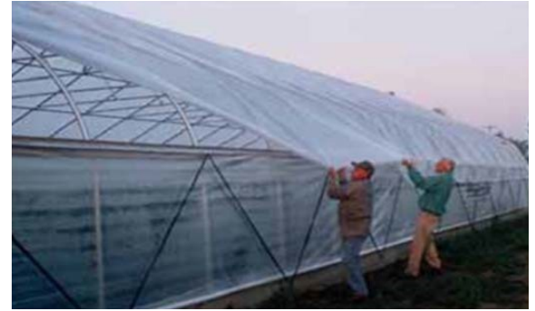
Figure 27: Fastening plastic to hipboards.
