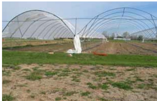
Figure 32: To apply plastic, the bundles are placed in the troughs between bays then pushed to the peak, unfolded, and secured in place with ropes (left). At the end of the growing season, plastic covers on multi-bay high tunnels are bundled and secured between the bays as shown (right). This method prevents damage to the film during the winter months when no crops are grown inside.
