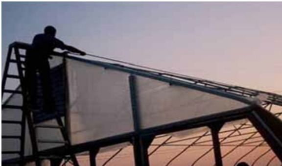
Figure 26: Installing the plastic film to the end wall of a high tunnel.
