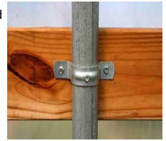
Figure 16: Fastening batten board to frame.
