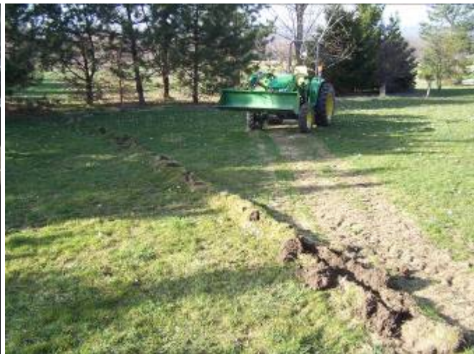
Trench for supply line
