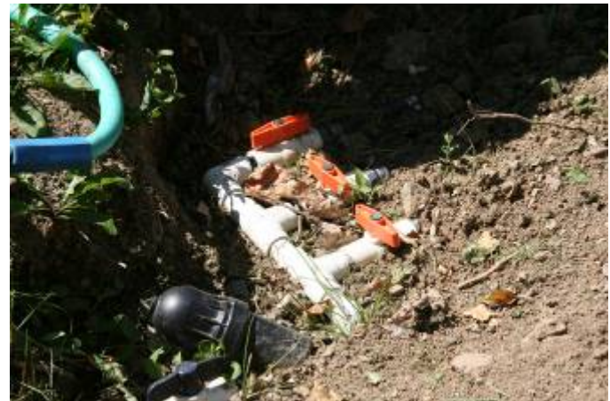
Hand valves for irrigation zones
