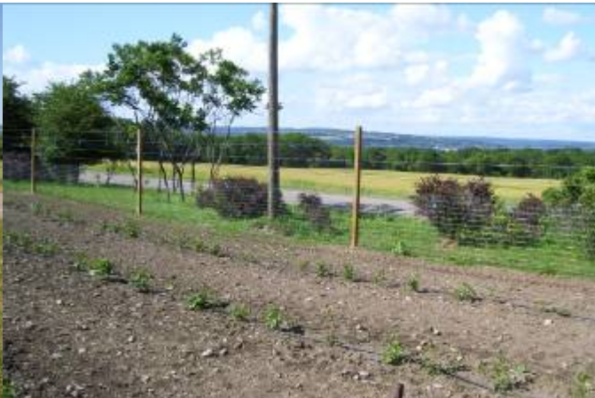
Welded wire fencing lines the bottom of the deer fence.
