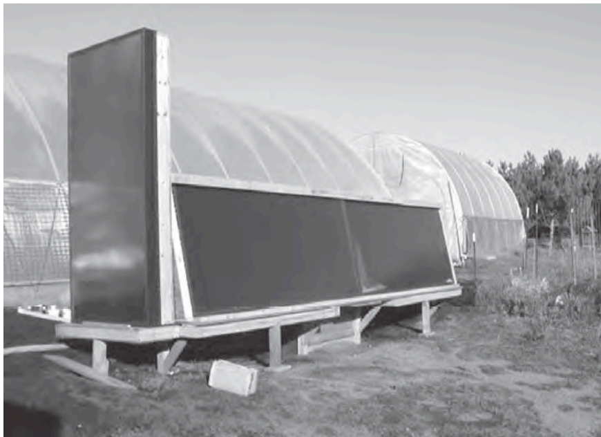
Figure 2. Solar panels on the south and east side of the high tunnel.
