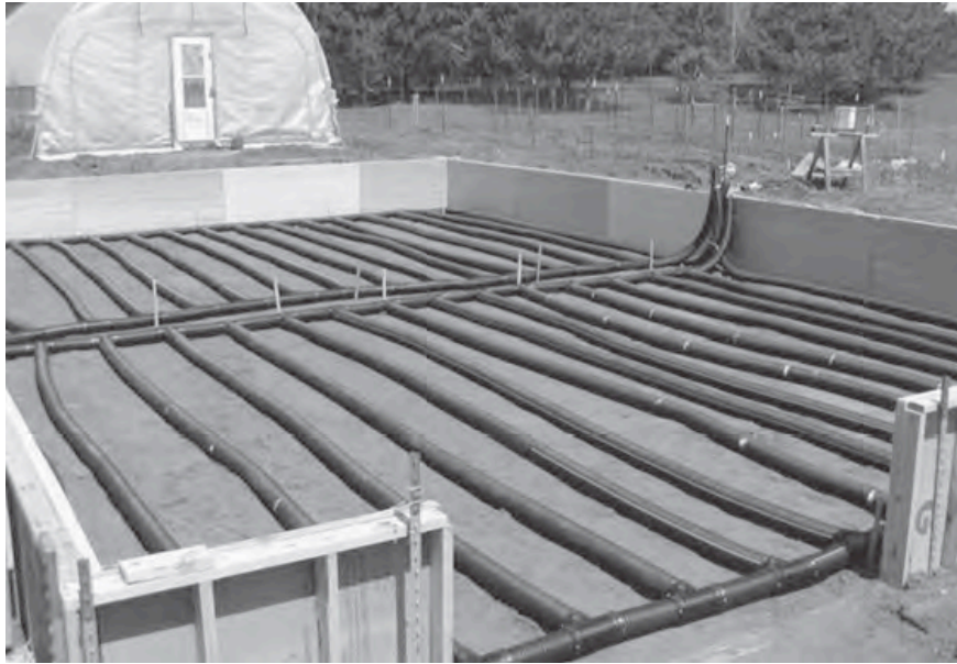
Figure 1. The lowest layer of tile line with the traditional high tunnel in the back ground.
