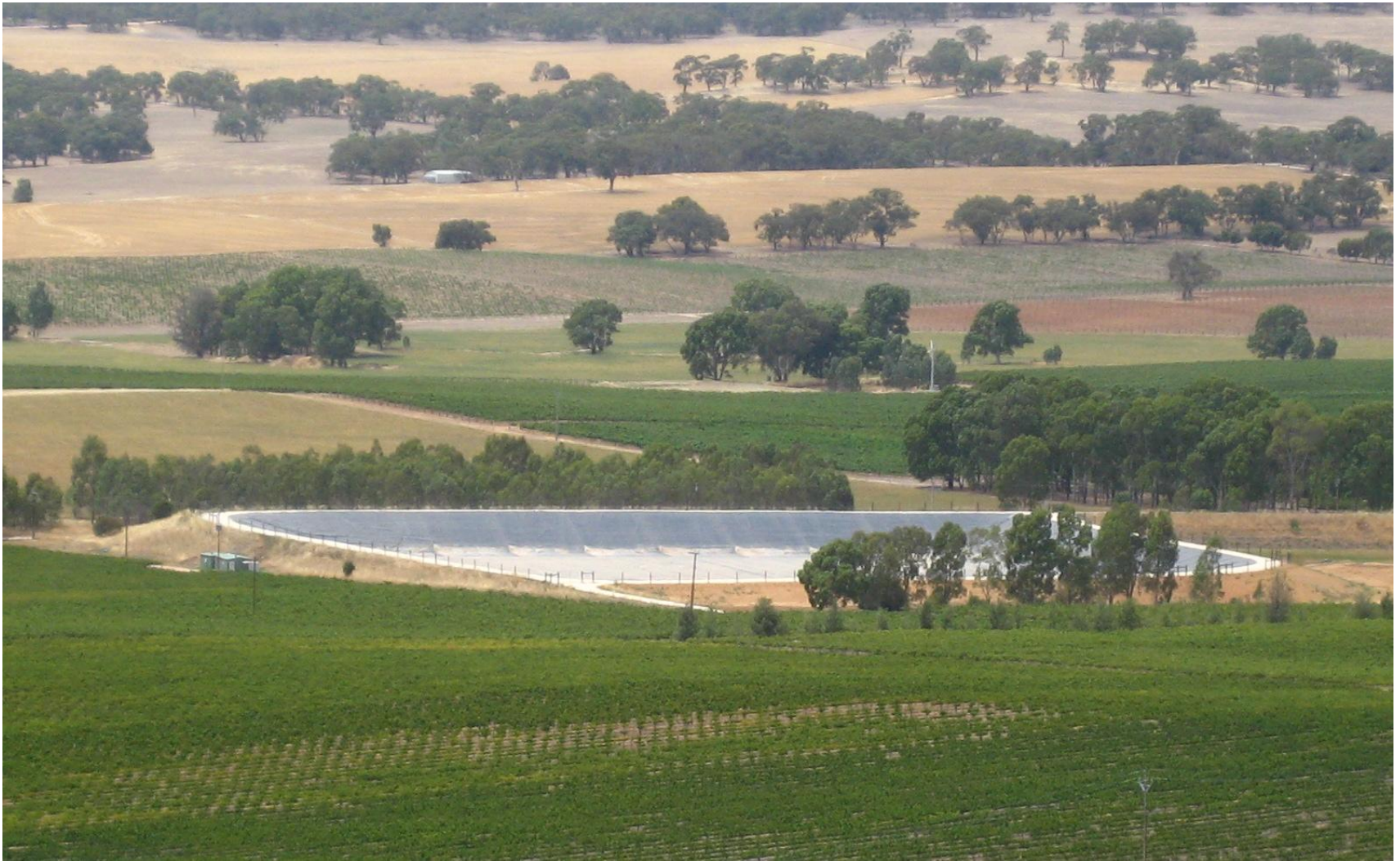
Inflatable Dam, Penfolds, Clare Valley
